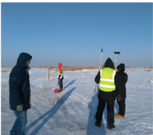
The frontline construction team works on snow-covered land
