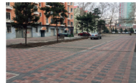
Water permeable pavement in the sponge city neighborhood
