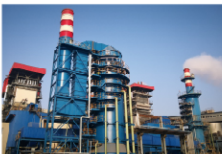
The ultra-low emissions renovation project at Qingdao Longfa Thermal Power Plant
