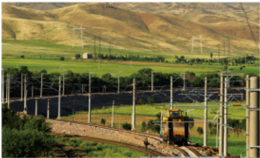
The electrification project of the Marokand (Samarkand)-Karshi railway line in Uzbekistan
