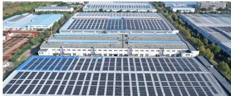
The 18MWp distributed PV power plant of Genertec Dalian Machine Tool reduces CO<sub>2</sub> emissions by approximately 20,700 tons per year
